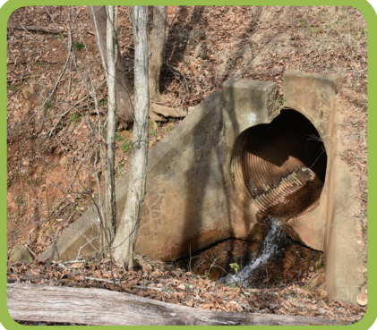
An existing stormwater outfall from Interstate 64 near the Old Mills Trail. This type of facility is discouraged.
